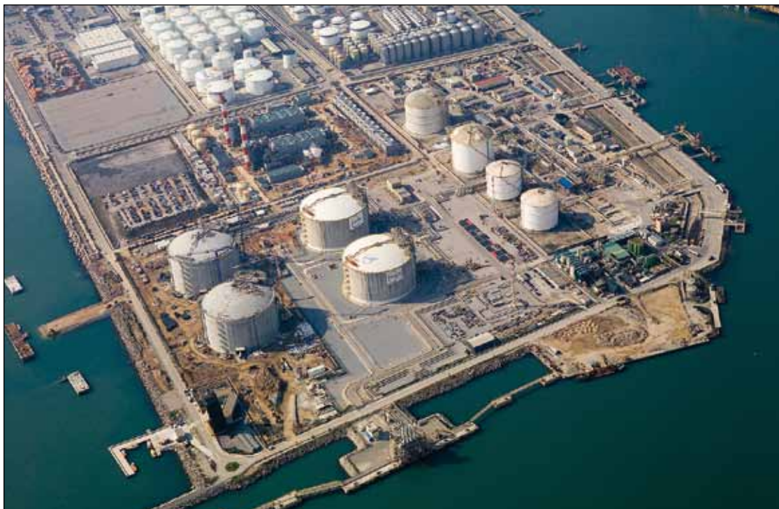
PGC A's first meeting was held in Barcelona where delegates had a technical tour to the Enagás regasification terminal.
